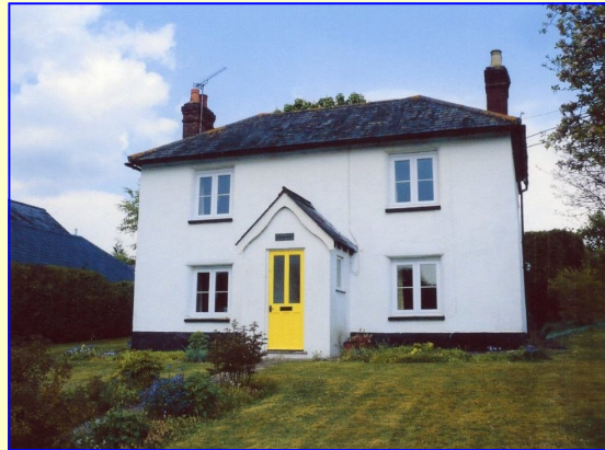
A typical Land-court house
